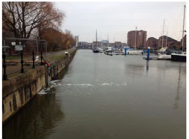
Photo 4: Discharge point, 12 Dec 13, showing wider view of Railway Dock
