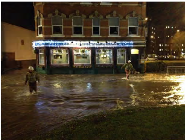
Photo 11: Flooding caused by tidal surge, looking W across Commercial Road
